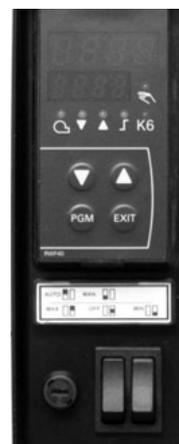
Fig. 47 - Burner modulator
