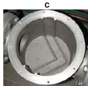
**Inspection and replacement of the MULTIBLOC DUNGS MBC..SE filter (Threaded valves group)**
